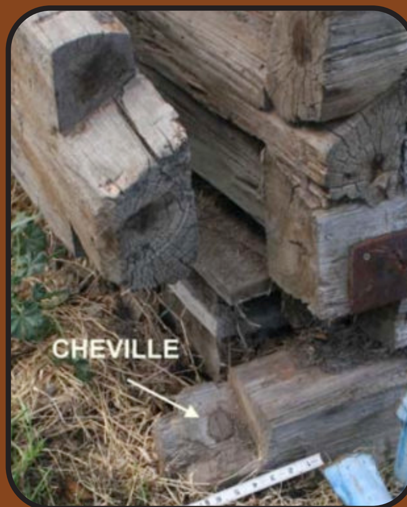
Left : Note the cheville or dowel pin holding the first log to the sill.
